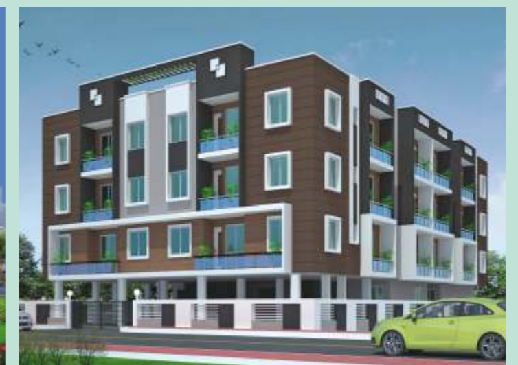
Lotus Tower Shivpuri, Patna (Running Project)
